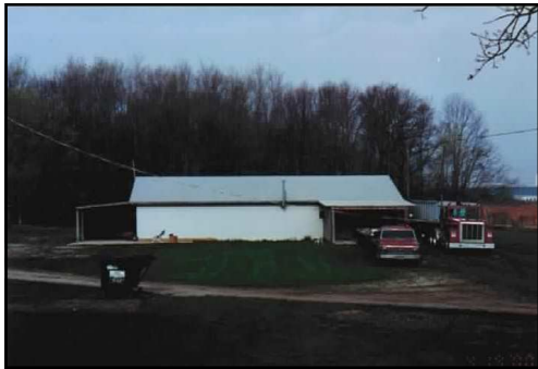
Construction begins on the original barn.
