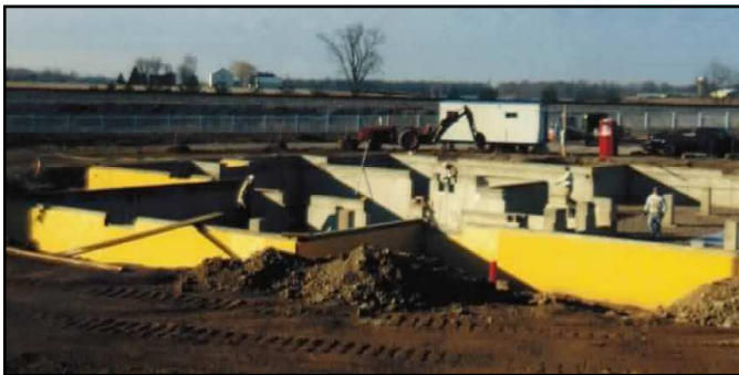
The foundation of the Victorian Farmhouse
