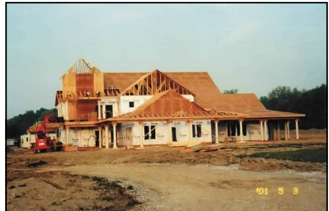
The Victorian Farmhouse takes shape.
