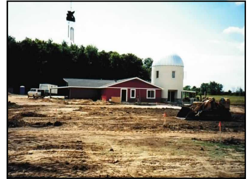
The Red Barn with silo in place.
